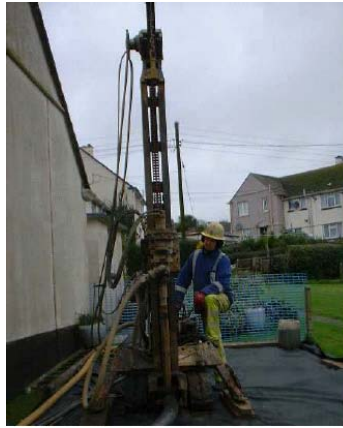
Drilling rig beginning a new borehole
